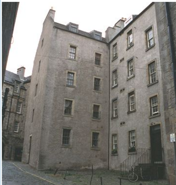
Edinburgh Charity Poorhouse site former east wing, 2001.
