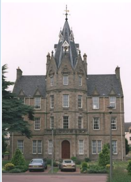
Edinburgh Craiglockhart Poorhouse central block from the south, 2001.
