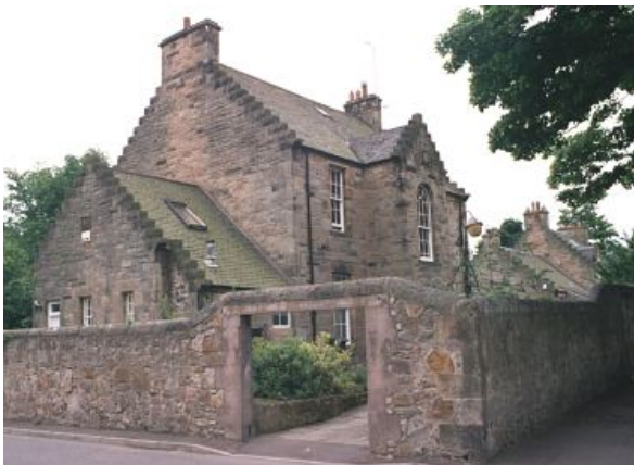
Edinburgh Craiglockhart Poorhouse governor's house from the north-east, 2001. © Peter Higginbotham.
